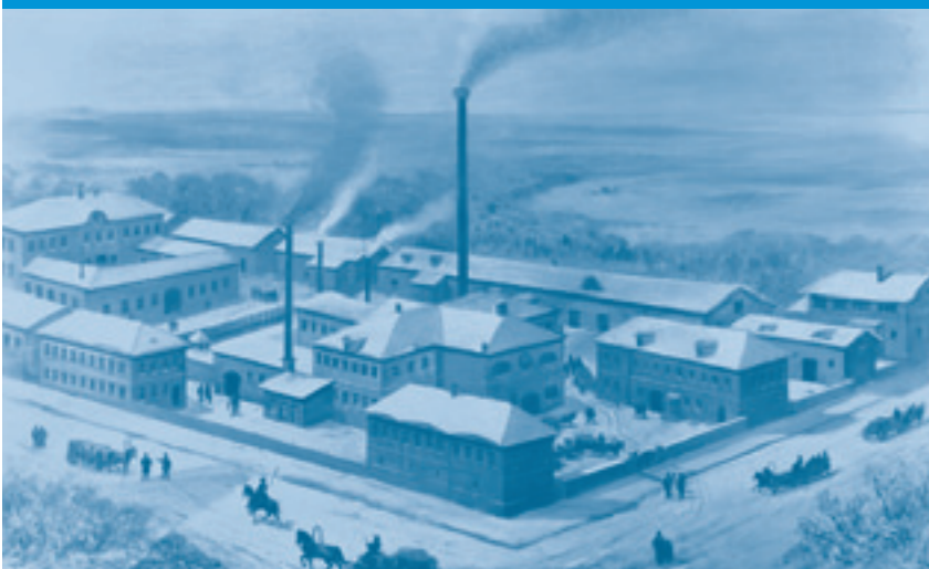
BASF's factory in Butirki near Moscow
