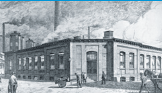
The company's first onsite medical clinic around 1914: The royal Bavarian medical superintendent Professor Koelsch hails it as a "remarkable facility with treatment, operating and X-ray rooms plus halls for therapeutic gymnastics and medical baths."
