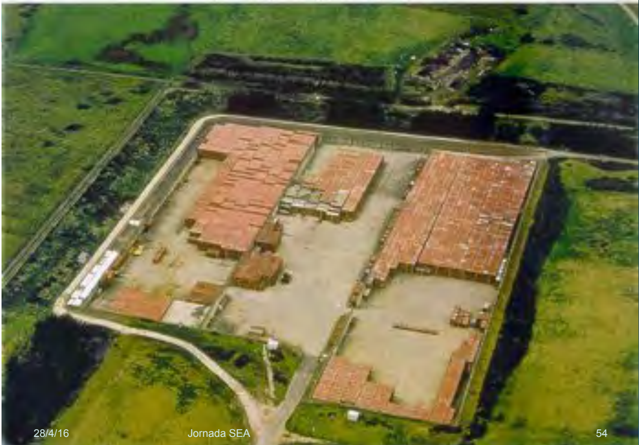
Figure 5-12: Aerial view of Urigg Low-Level Waste Site showing freight containers stacked in Vault 8
